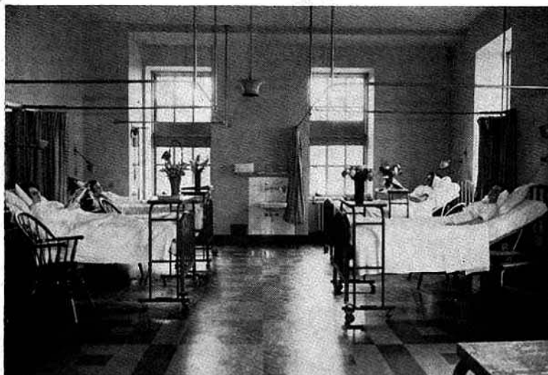
Fig. 2.—Photograph showing a typical four-bed ward.
